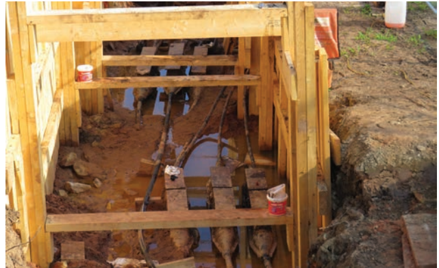
Figure 5. Photos of field joints being used to connect separate sections of cables together.
