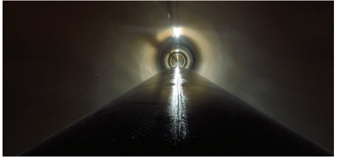
FIGURE 1. An inside view of the hyperloop test track.
